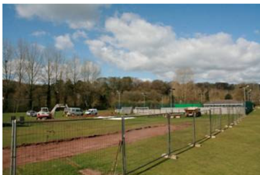
Ground works getting underway
